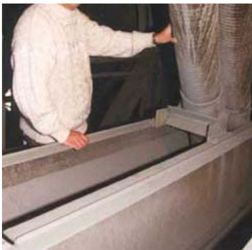
Lonmin R&D superintendent Craig Goodall demonstrates the use of flexible piping allowing simple reconnection to different cells along the bank to simultaneously produce high, medium and low grade PGM concentrates.
